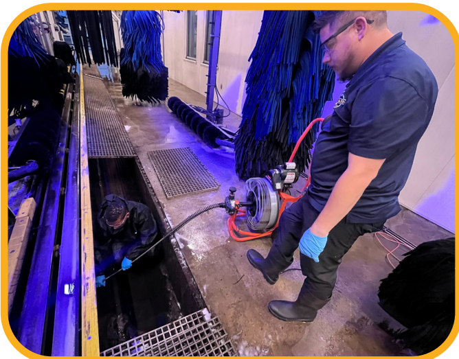
Regional Director Justin Sain (right) and Site Leader Jeremy Bratcher (left) snaking the drain at our Hughes location at 9:30 pm on a Friday night
